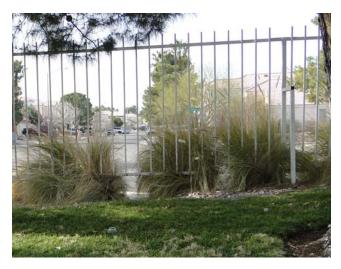
2014 - Fencing is in need of rust treatment and painting. A section of fencing atop a block wall surrounding a small greenbelt area at the intersection of Lady Lake and Fairvilla was painted in 2012. It appears that this fencing, due to deferred maintenance, may need some repair and extensive rust removal when painted.
